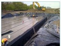
Underground Stormwater Management Chamber
